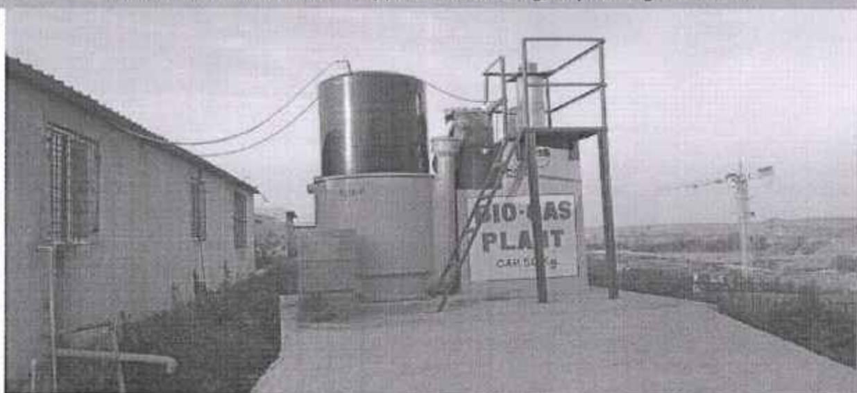
Bio-Gas Generation Plant – Approximate 100kg/day- College Canteen
